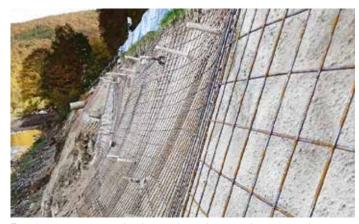
Reinforcement is in the form of two layers of steel mesh.
